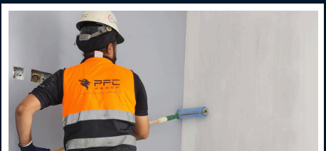
Corporate Office Renovation Works- EMAAR
