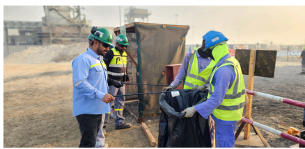
Enhancing Worksite Hygiene Through Cleanup Efforts
