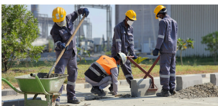
Kerbstone Installation Works- EMAAR
