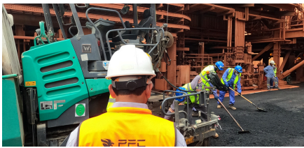
Infrastructure Construction- Al Taweelah Refinery
