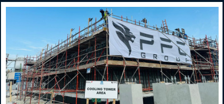
Construction of Cooling Tower- KEZAD
