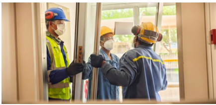
Corporate Office Renovation Works- EGA
