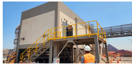
OBxR Sub Station Works- ATA
