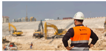
Construction of New Metro Line- RTA
