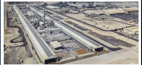
Casthouse Extension- EGA
