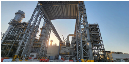
700T Structural Crane- EGA
