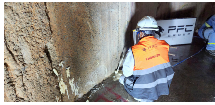
Rehabilitation of Casting Pits- Kezad
