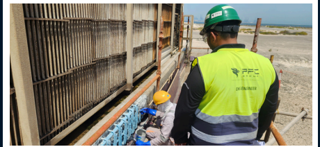
Concrete Rehabilitation Works- EGA
