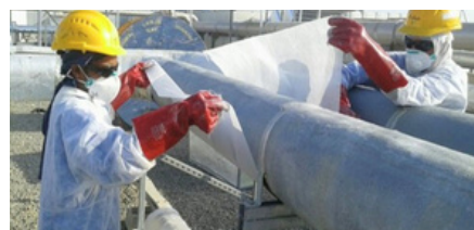
Glass Reinforced Plastic Works- Majid Al Futtaim
