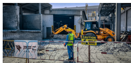
Industrial Floor Breaking Works- EGA
