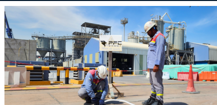
Joint Sealant Works- EGA
