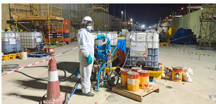
Foundation Strengthening Works- IKK Group
