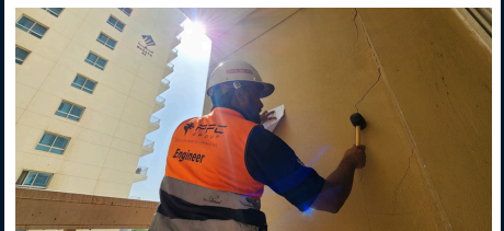
Surface Restoration Work- Al Mazaya
