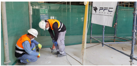
Utility Plant Crack Injection- AD Ports
