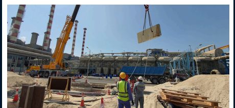
Structural Rehabilitation Works- DEWA
