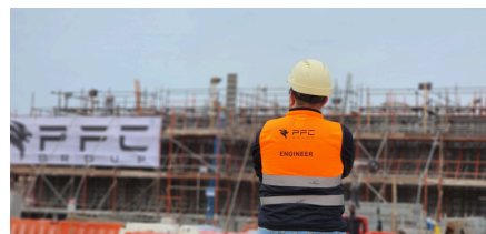
Rehabilitation of Water Tank- AD Ports
