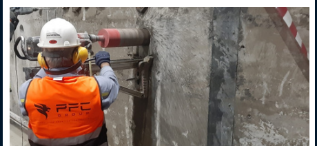
Concrete Coring Works- Jumeirah Group
