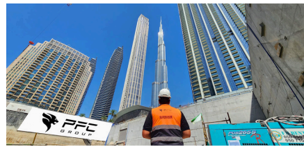
Residential Building Demolishing Works- Dubai Properties
