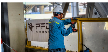
Fiber Reinforced Polymer Wall Replacement- EGA
